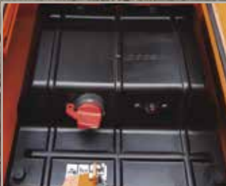
Battery cut-off switch
